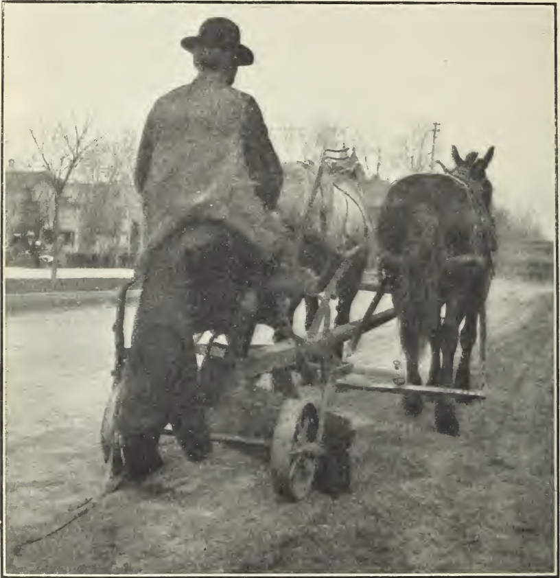
FIG. 10.—Type of horse-drawn road grader.
